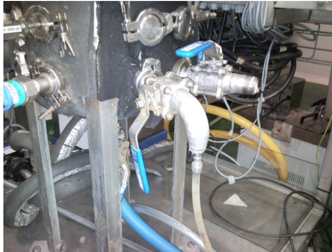
Picture 1- influent tank sampling port
