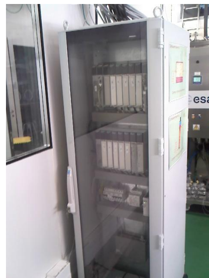
Figure 8. CI PLC cabinet: initial configuration (left) and after refurbishment (right)
