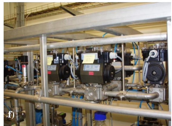
Figure 9. Some details of hardware modifications on CI filtration unit: a) 3-way ball valves in filtrate line; b) 3-way valves and deadlegs in retentate; c) distribution of valves in retentate pipelines; d) N2 inlet in filtrate tank; e) screwed sensor and drain connections in filtrate tank; f) cleaning and steam 3-way valves
