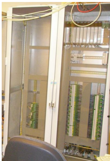
Figure 8. CI PLC cabinet: initial configuration (left) and after refurbishment (right)
