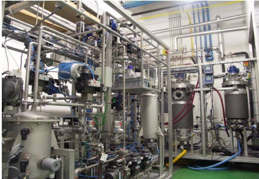
Figure 4. Final CI configuration in MPP after installation
