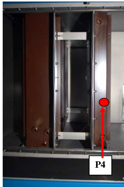
Figure 8 Pressure probe between the heater and the cooler
