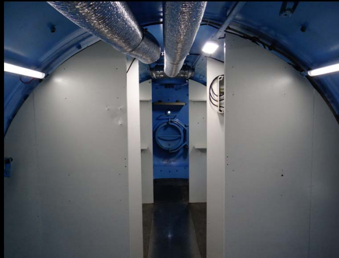
Forward hatch of the habitat
