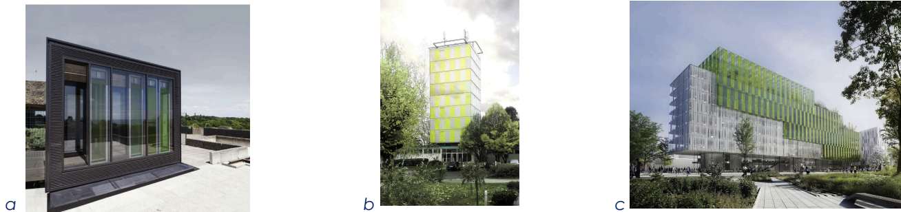
Figure – facade photobioreactors a) SymbIO-BOX in Saint-Nazaire, b) CSTB building in Champs-sur-Marne (2016), c) Future building ALGUESENS project, Paris
