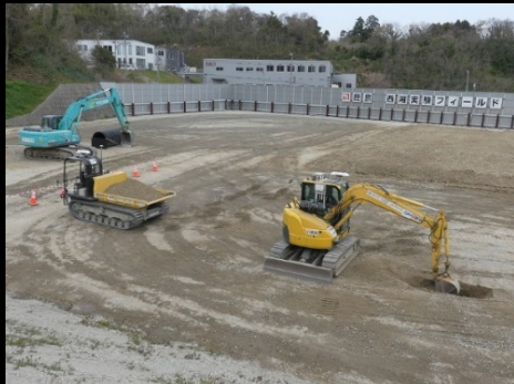
Innovative remote construction system
