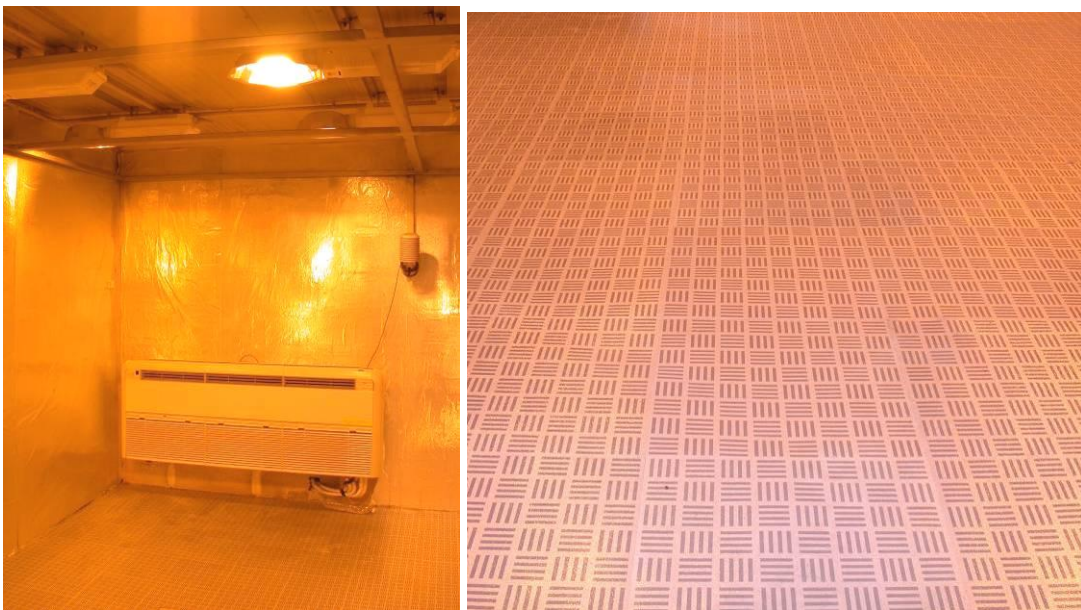
Fig. 56 Air conditioning system in the growth chamber and reflective film on the floor.
