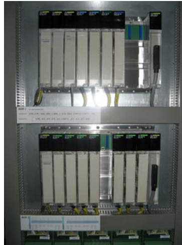
Figure 5-6 PLC assembly on backpanels
